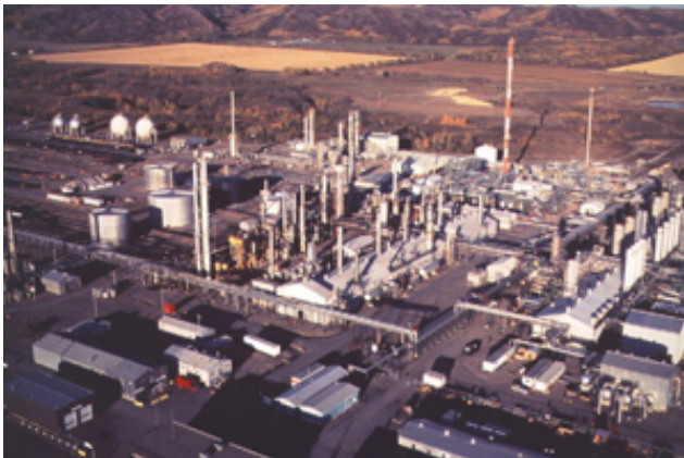
A Natural Gas Processing Plant
